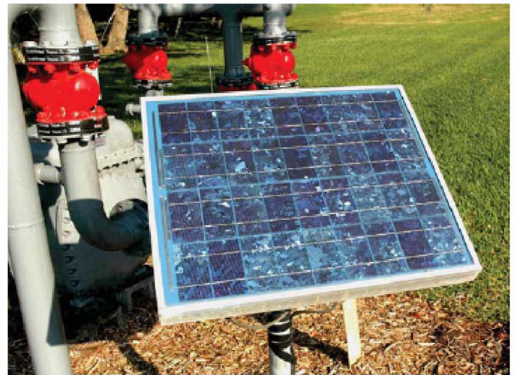
Figure 2. Small solar panels can be used to power pumping stations in greenhouse operations.
