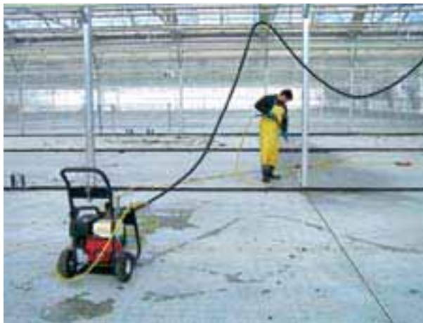
Figure 1. Cleaning, then disinfesting concrete floor joints and cracks is critical for minimizing potential disease problems in recirculating systems like flood floors.
